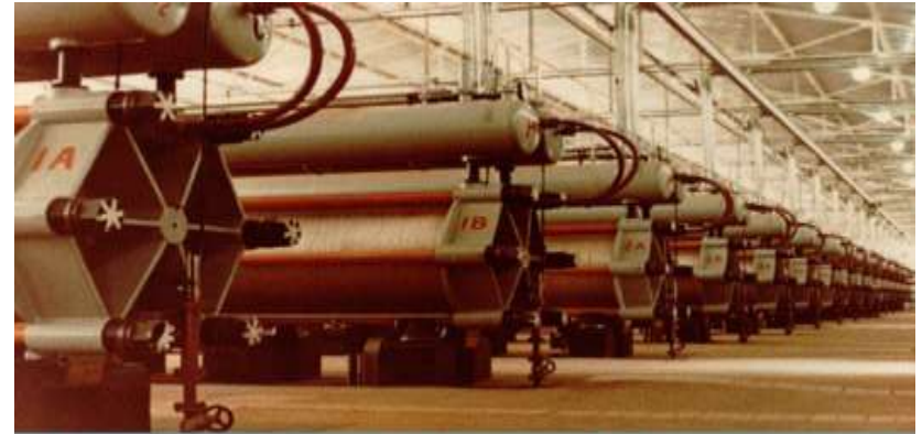
21'000 Nm 3 /h H 2 electrolysis plant
